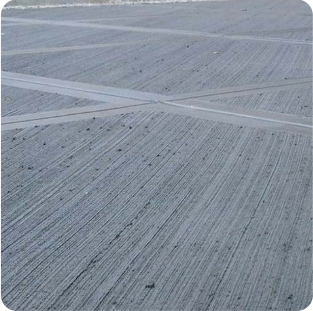
Brushed Concrete Footpath
